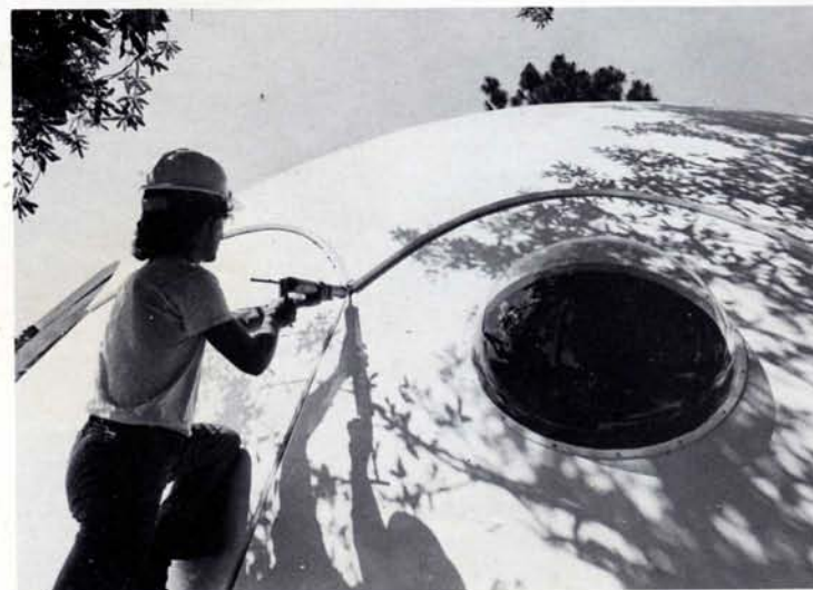
Top left: Fiberglass panels are coated prior to installation. Left and above: Mr. Yacaboni's son installs a Tested and Approved Sealant manufactured by DAP, Inc.
